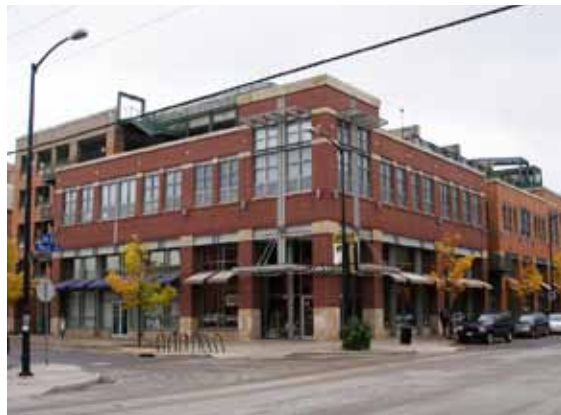
Portions of parking structures facing public areas should relate well to human scale, complement the character of adjacent buildings, and incorporate visually attractive elements.
