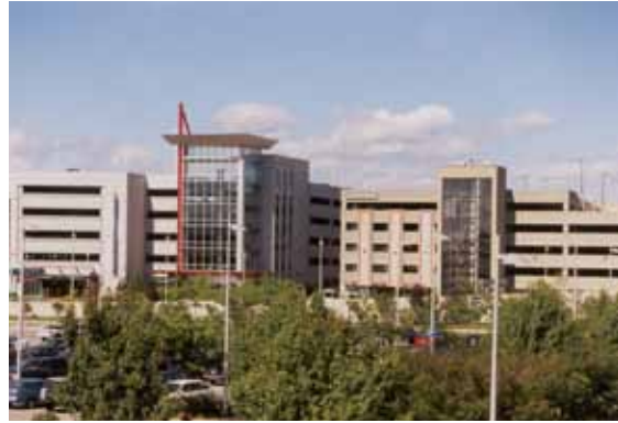
New parking structures with space for nearly 2,100 vehicles were built to serve the Bruce Sundlun terminal.
