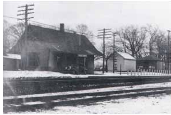
The Hillsgrove Station, pictured in this historic photo, once served residential and industrial uses around today's Redevelopment District.
